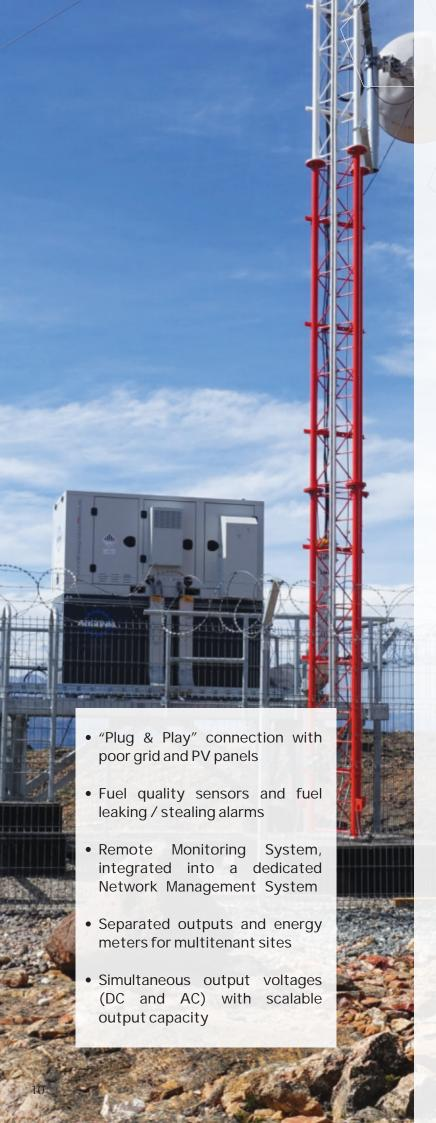
For the BTS power supply applications, Ausonia has developed a complete family of **HIGH EFFICIENCY DC SOLUTIONS**, representing the latest variable speed power generation technology now available in the market and offering the right balance among lowering CO<sub>2</sub> emissions, reducing operational costs and enhancing the overall fleet efficiency, with a specific fuel consumption rate of only **0,4 l/kWh**.
